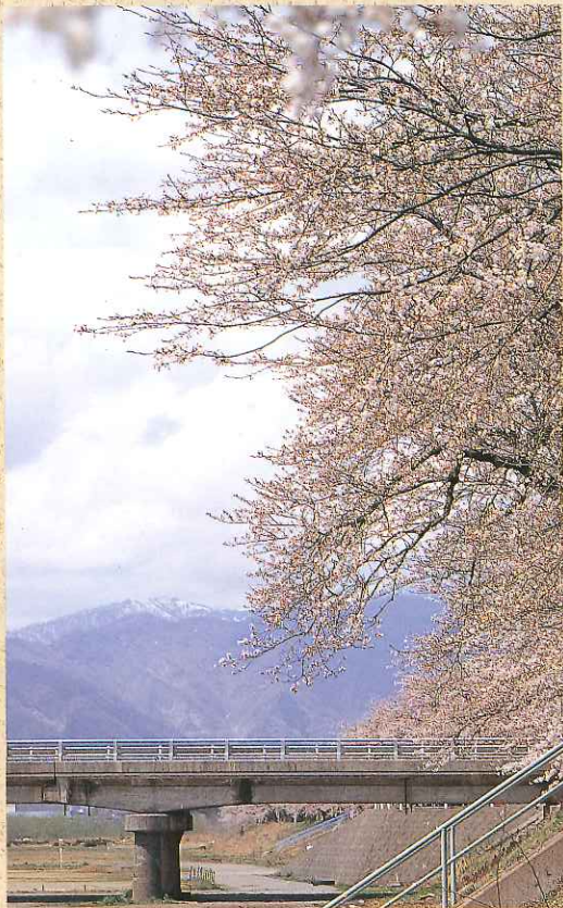
勝山橋 Katsuyama Bridge
